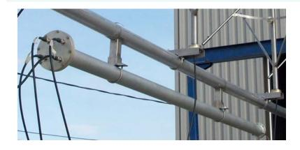
Pictured to the left is a pancake style power divider. This one is for FM and has a 3-1/8" EIA input. The divider is 10 feet long.
